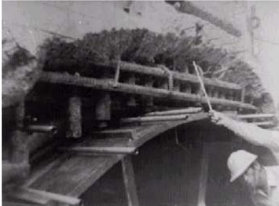
Figure 2.12. An overhead repair with congested reinforcement where the need for consolidation of preplaced coarse aggregate is unavoidable
